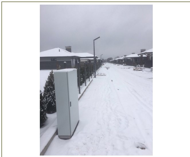
Fig. 4 The smart meters is in the metal cases along the street without external antennas. Distance between metal boxes is 40-50 meters.
