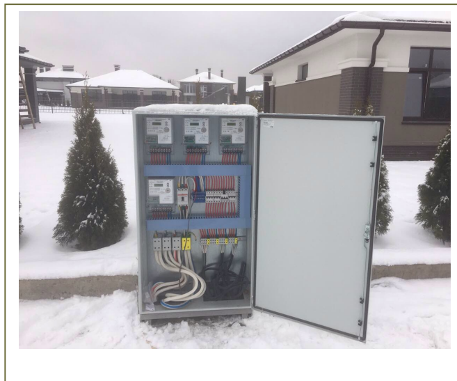
Fig. 5 In the metal box is 4 smart meters with integrated Embee modems. Modems have chip antennas. Output power of modems are 100mW.
