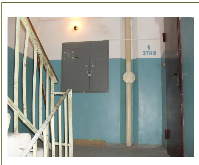
Fig. 6 The smart meters install in metal box in ferroconcrete wall at 5 floors (4 porches).
